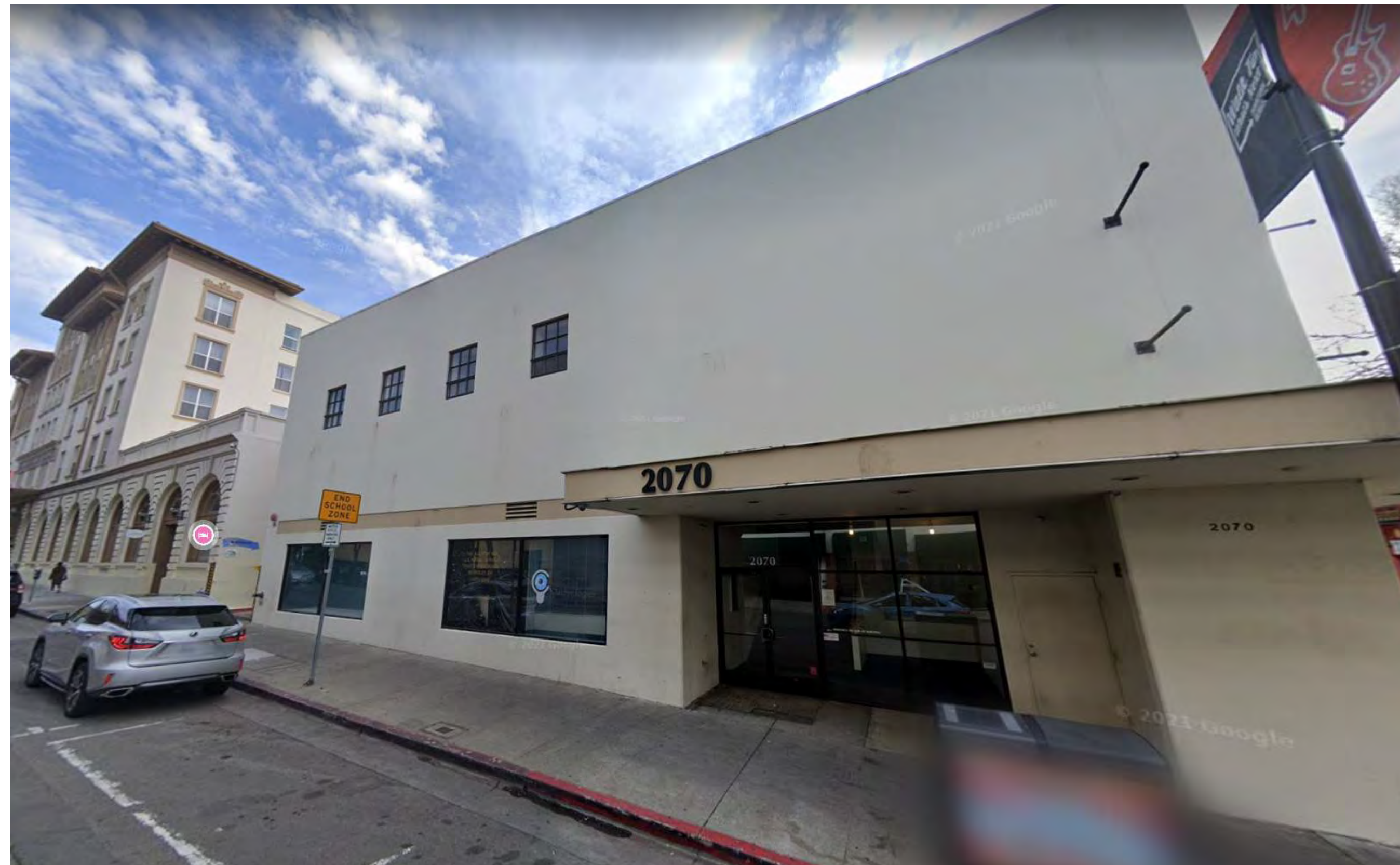
1 SITE PHOTO - ALLSTON WAY FACADE A0-002 12" = 1'-0"
