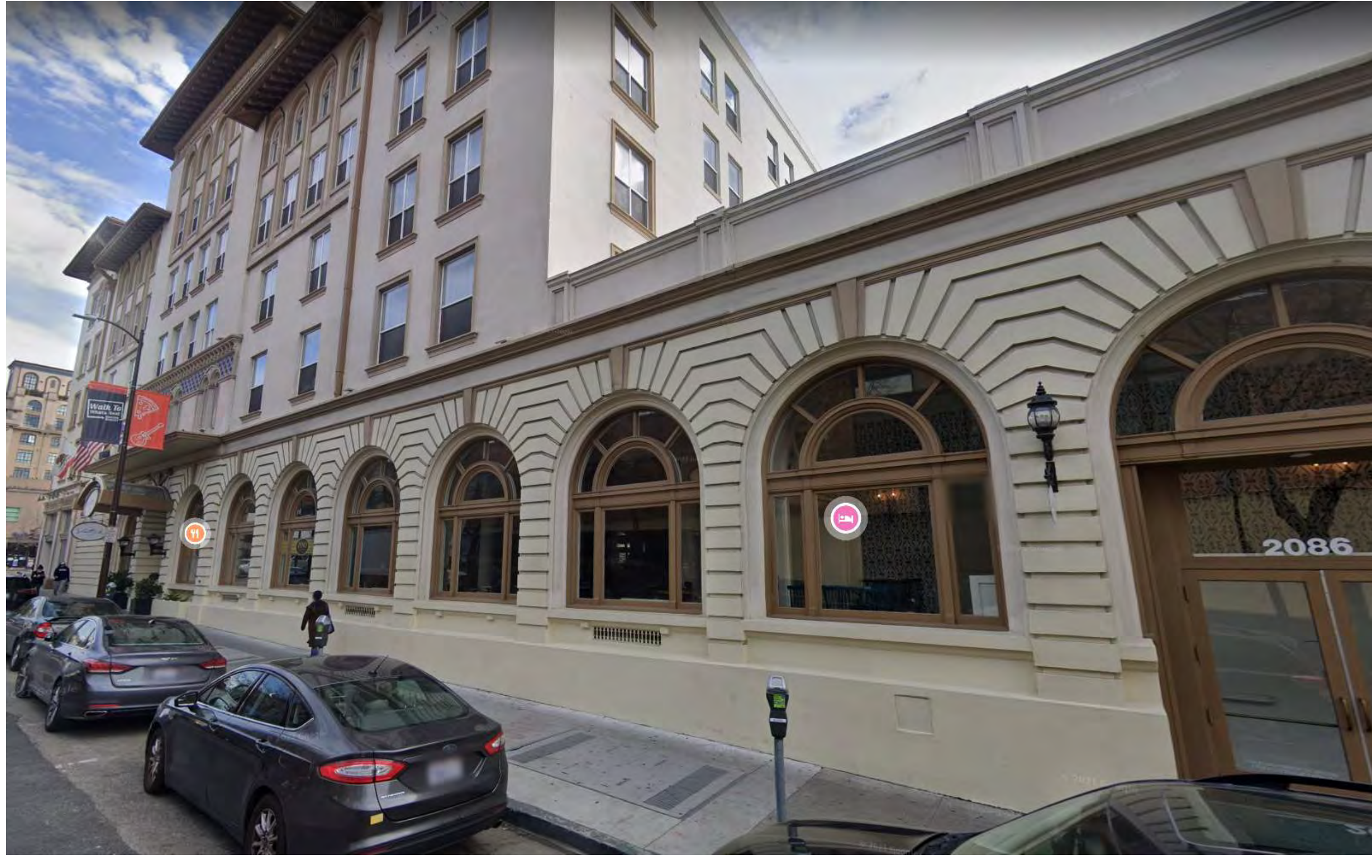
1 SITE PHOTO - ALLSTON WAY - EXISTING HOTEL A0-003 12" = 1'-0"
