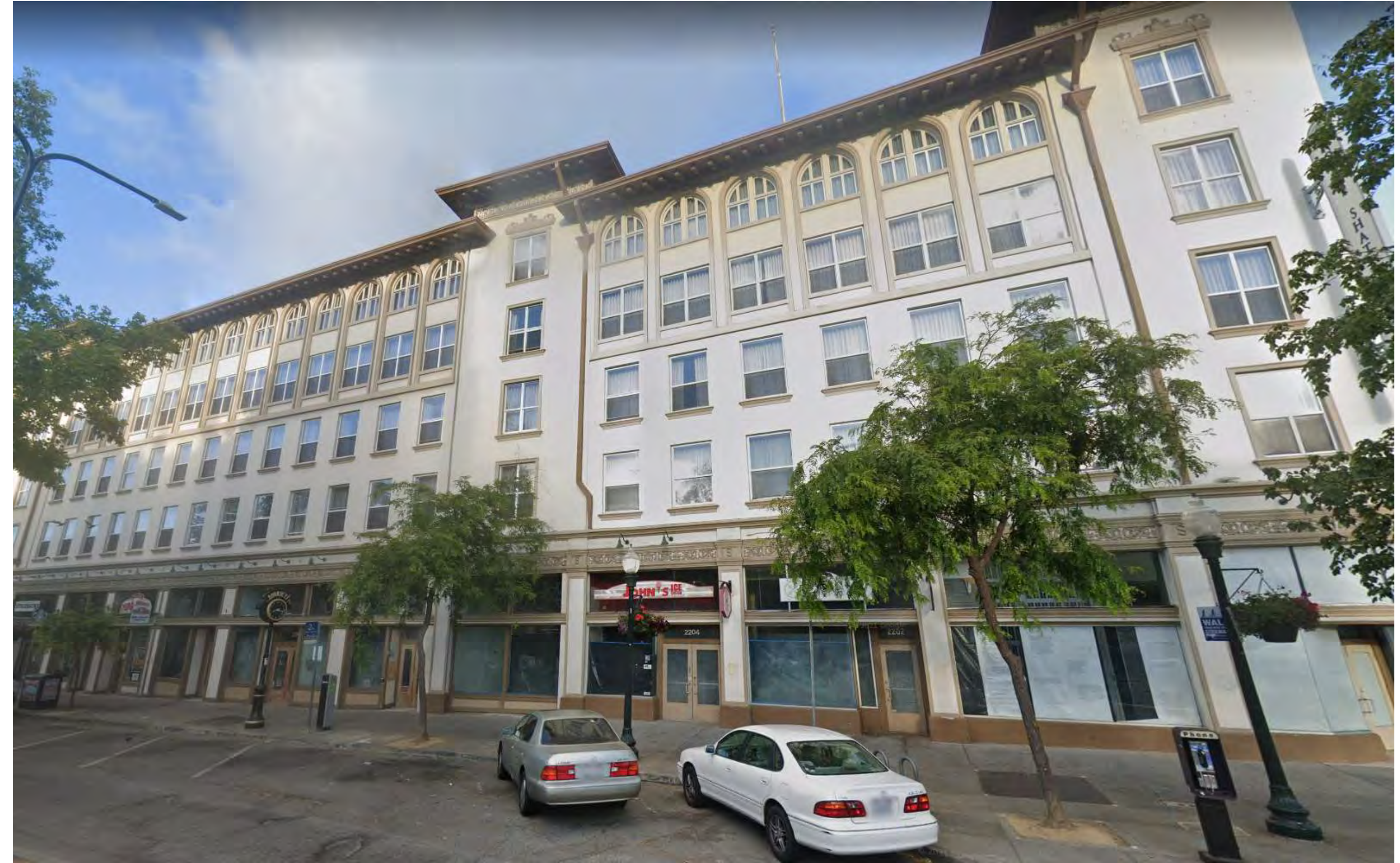
2 SITE PHOTO - SHATTUCK AVE - EXISTING HOTEL A0-003 12" = 1'-0"
