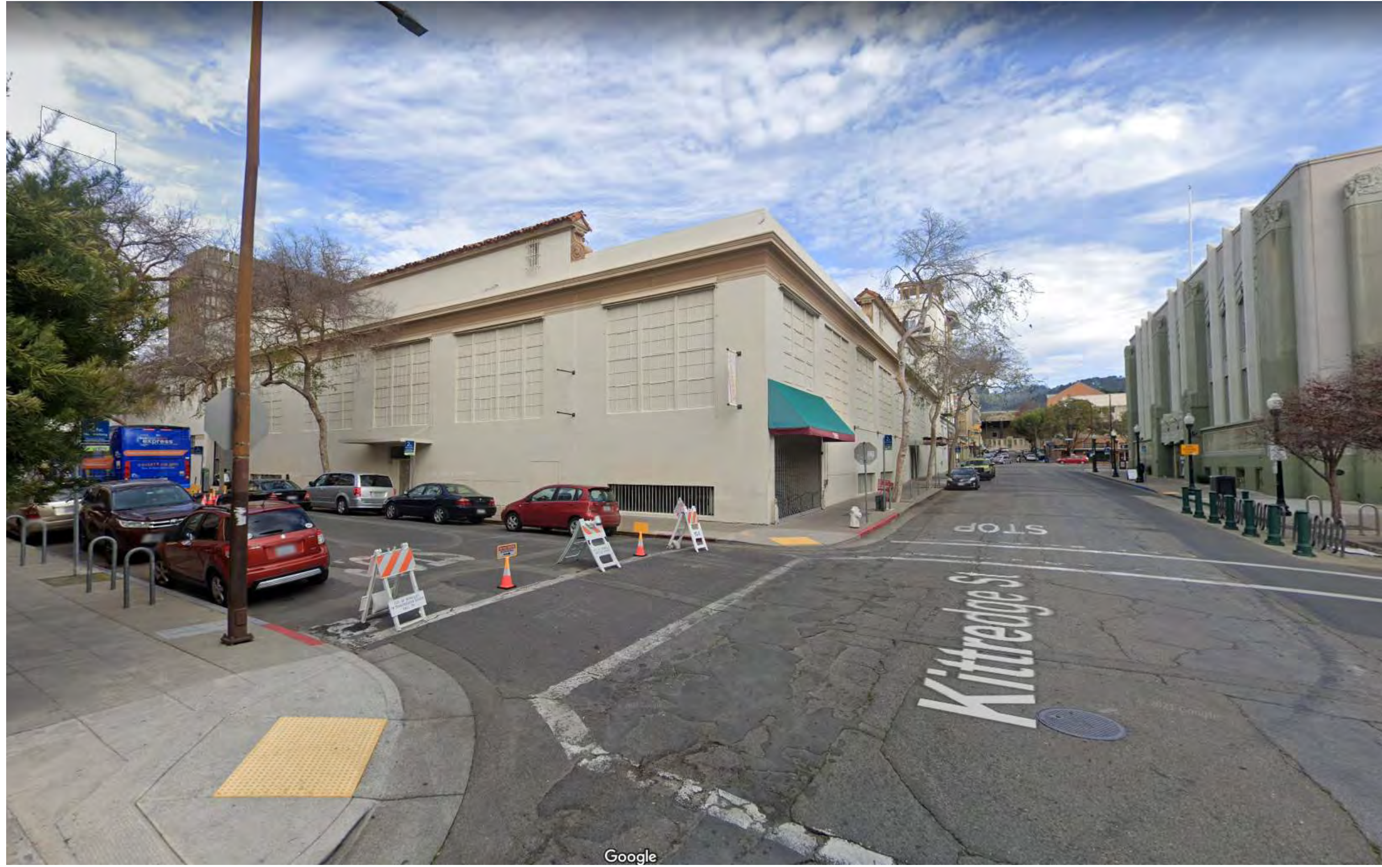
1 SITE PHOTO - KITTREDGE ST AND HAROLD WAY - LOOKING EAST A0-001 12" = 1'-0"
